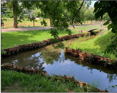
Fig. 1. The banks of the water gloss in the Alexandru Buia Botanical Garden from Craiova, reinforced with wooden pillars and reeds
